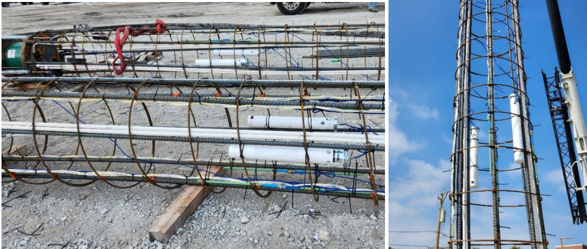
Fig. 4. Photographs of the Instrumented Reinforcing Cage
