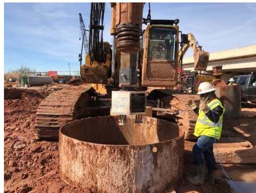
Figure 13 SQUID™ mounted on the Kelly bar (left) and 1 ton beam (right) at the construction site
