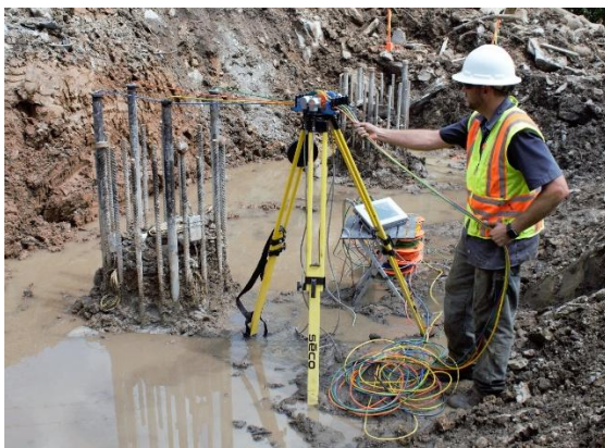
Figure 18 Access tubes installed on a foundation pile
