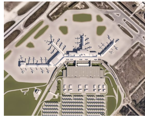
SW Florida International Airport – Expansion Arial View Concourse E
