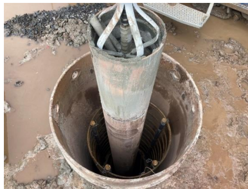
Fig. 5. Composite caisson-micropile prior to concrete placement.
