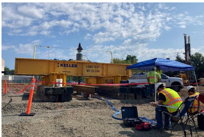
Fig. 1. Micropile Tension Test Setup (Test #1).
