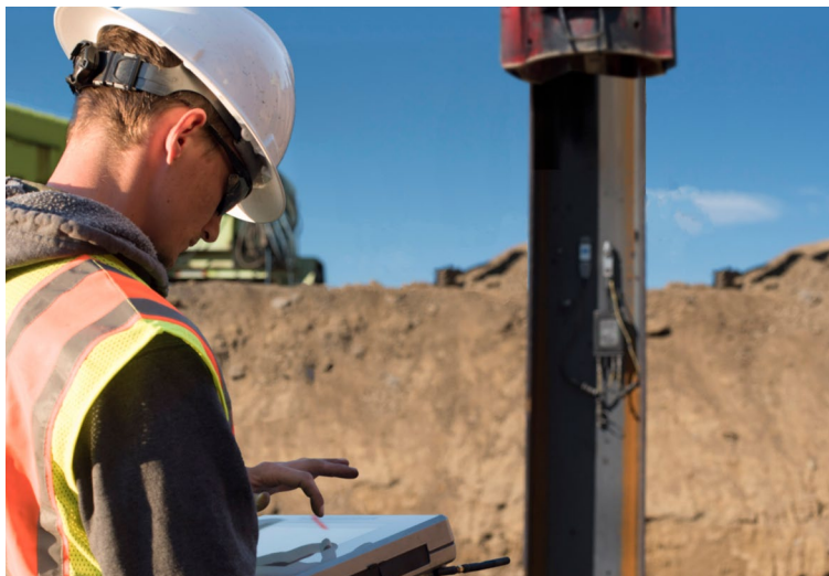
Figure 2. Pile Driving Analyzer® Monitoring H-Pile Installation
