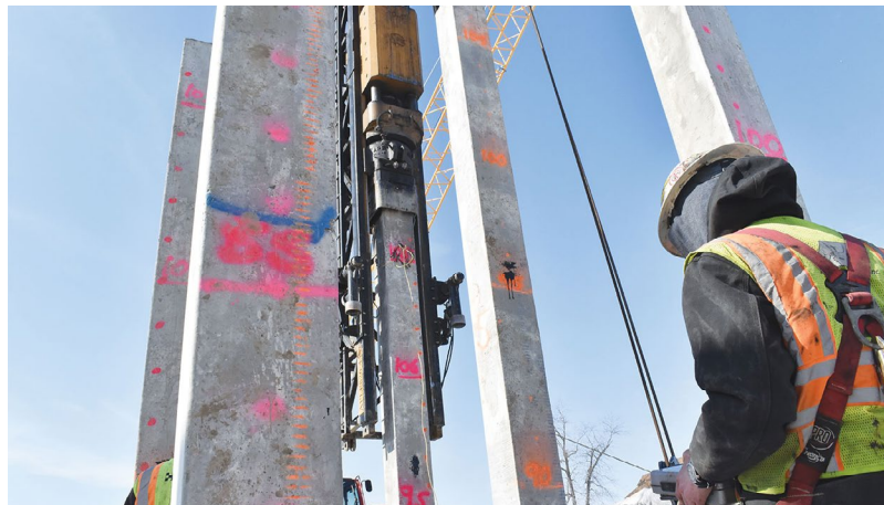
Figure 1. Using the Pile Driving Analyzer® to Monitor Concrete Pile Installation
