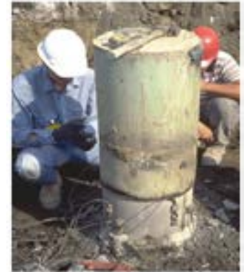
Figure 2. Side-Mounted Strain Transducer on pile-top build-up
