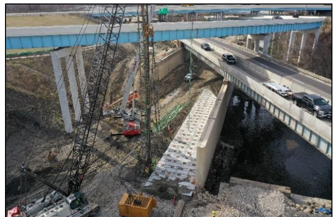
Photo 1: Phase 3 (Initial) ACIP Installation
