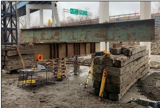
Photo 6: Static Load Test Set-up
