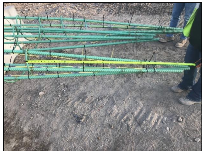
Photo 5: TIP instrumentation of rebar cage taper at bottom
