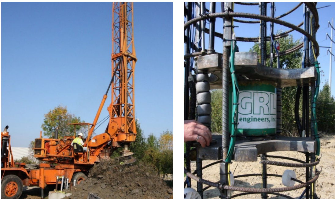
Fig 1. Drill rig and 300-ton bi-directional cell in cage for 2017 conventional BDLT
