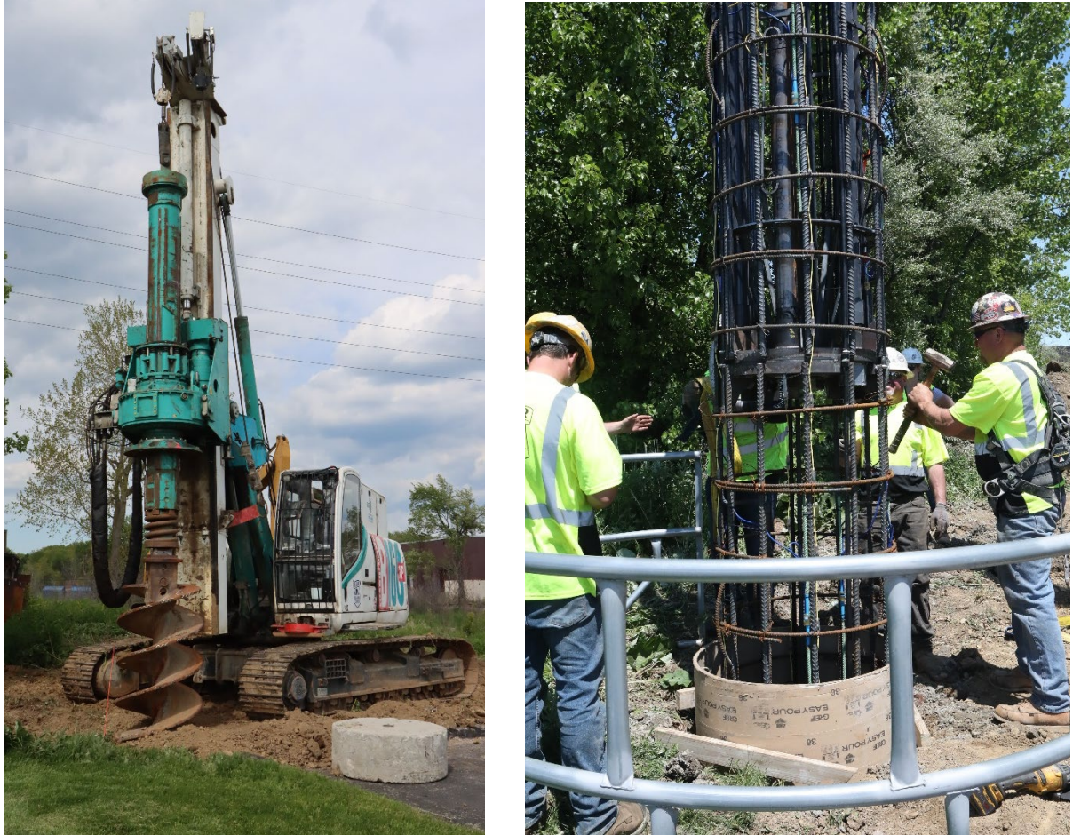
Fig 2. Drill rig and bearing plate assembly in cage for 2021 TLBT
