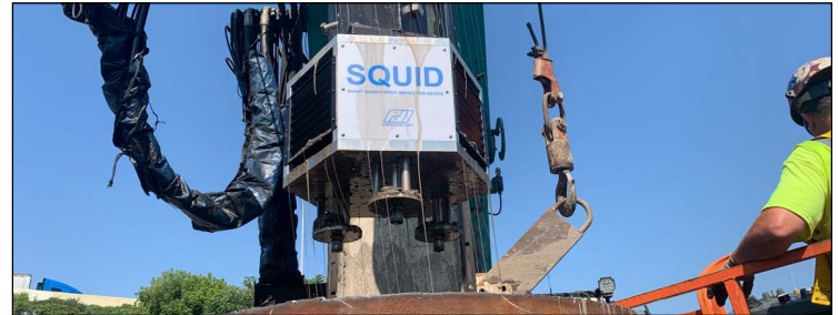
Image 2. Shaft Quantitative Inspection Device (SQUID) descending from drilled shaft
