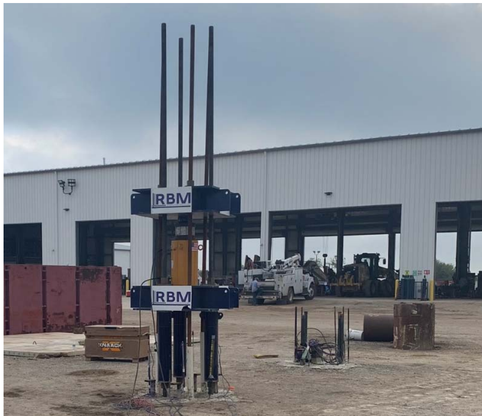
Figure 8. Finalized TLBT assembly immediately prior to testing
