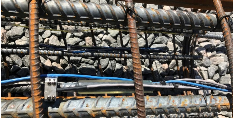
Figure 6: Resistive strain sensor and accelerometer are attached onto the reinforcement cage.
