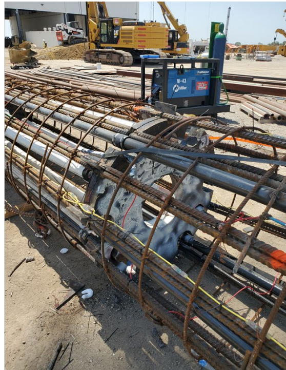
Fig. 3b. TLBT bearing plates in cage.
