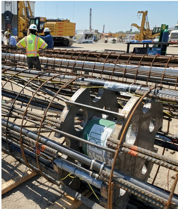
Fig. 3a. 500-ton BDLT jack assembly in cage.
