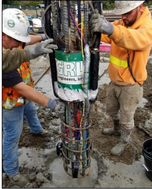
**Figure 3. BDSLT Test Pile TDDP-1 completed jack assembly and instrumented reinforcing cage.**
