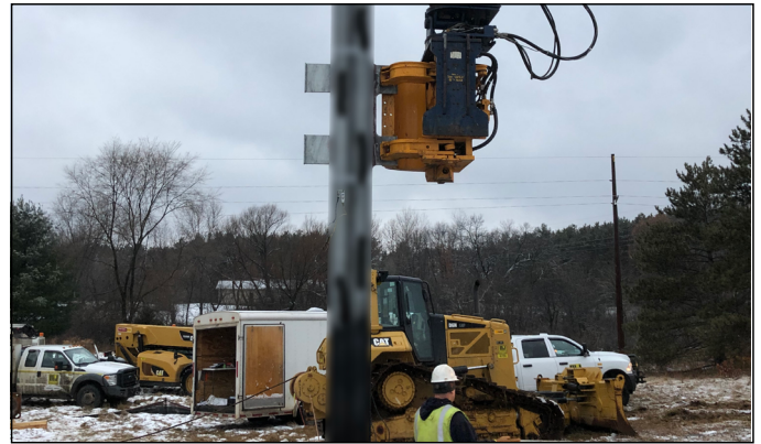
Pile Driving with a Vibratory Hammer
