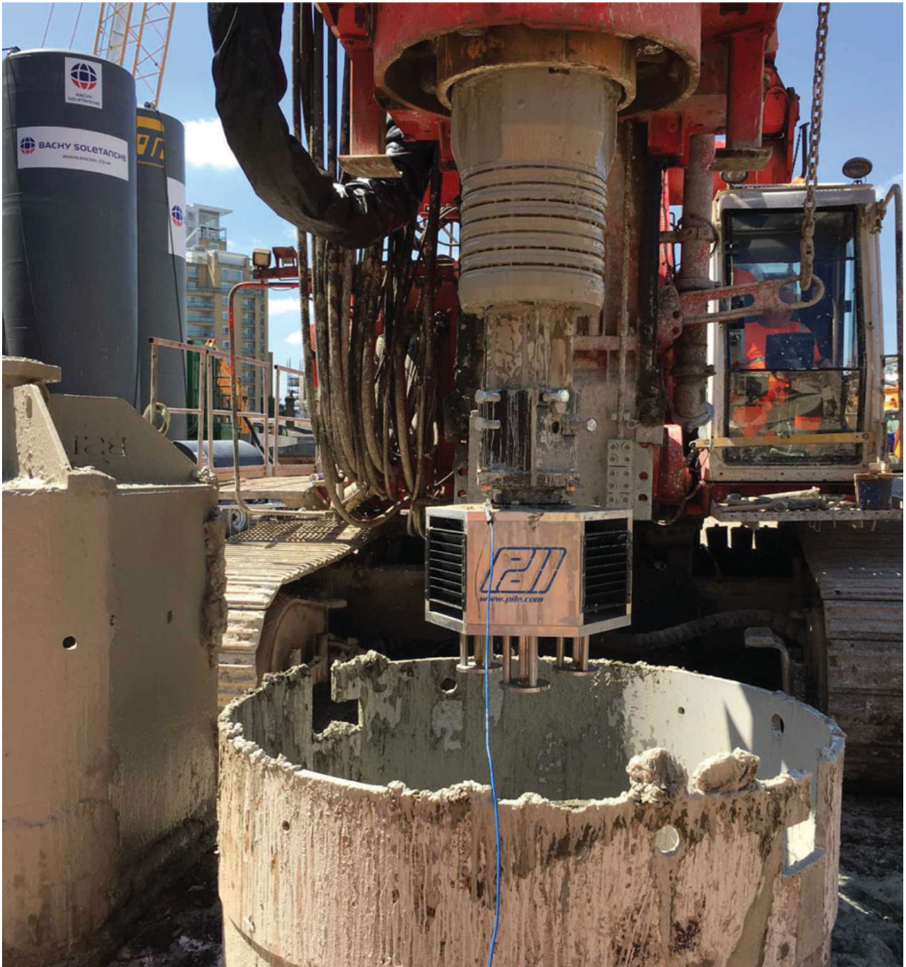
SQUID TESTING FOR A 72-IN DIAMETER DRILLED SHAFT
