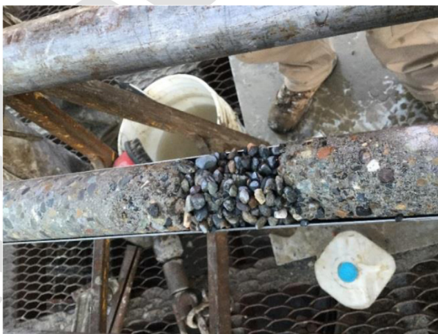
FIG. 8 Coring results in a defective drilled shaft.
