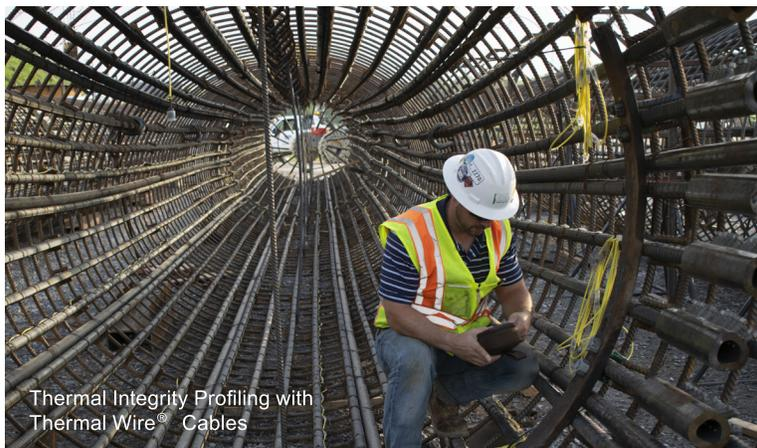
Thermal Integrity Profiling with Thermal Wire® Cables
