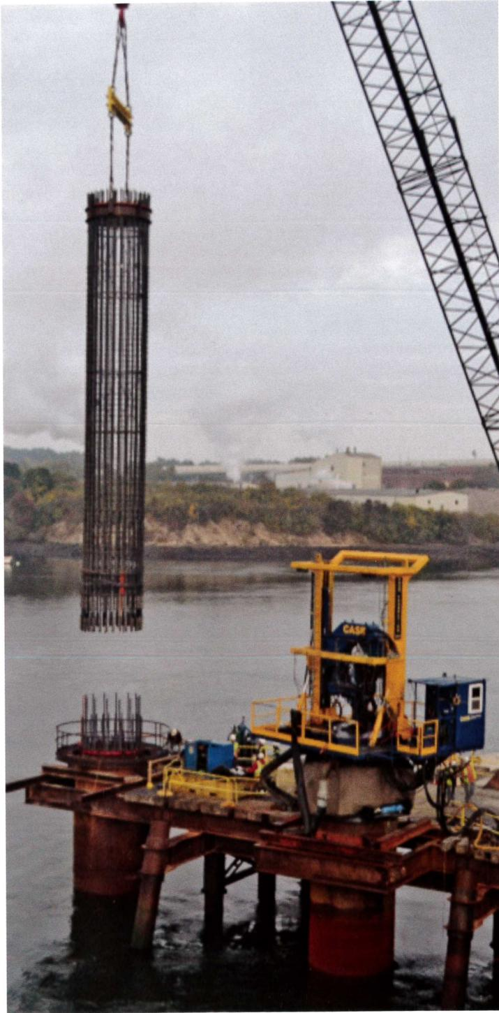
Figure 11: Reinforcing Steel Cage Placement.
