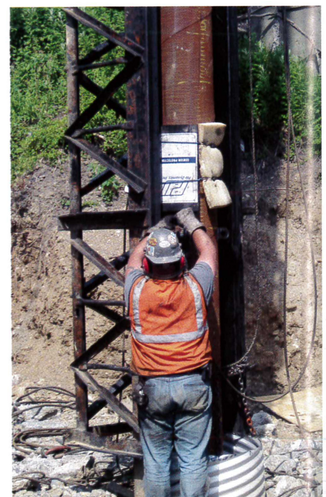
Sensors being installed on friction pile
