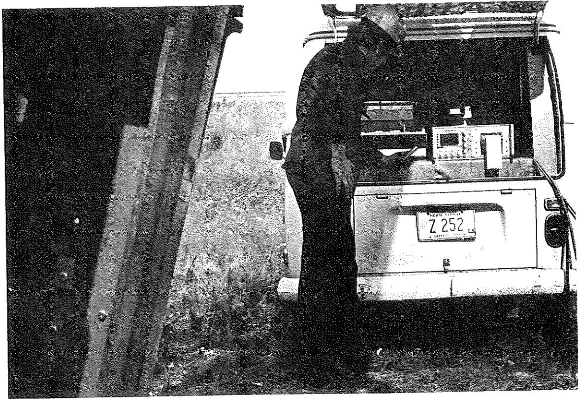
FIGURE 3 Case Method Pile Driving Analyzer and recording system with transducers on the pile (foreground left)
